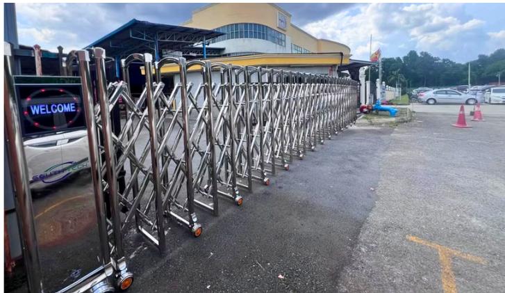
Wipro Warehouse Kajang
