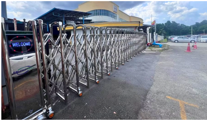
Wipro Warehouse Kajang
