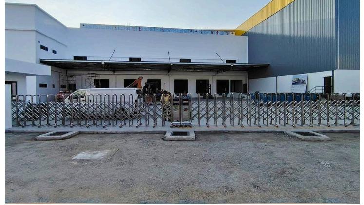
DHL Warehouse Penang
